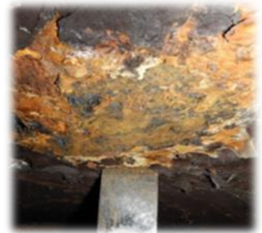
Corroded Pipe
