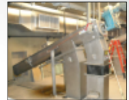
Shaftless Screw Conveyors
