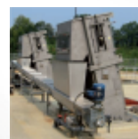
Chain Driven Multi Rake Bar Screen
