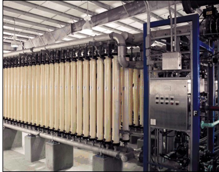
Figure 5-3. Full-scale Pall MF system (Source: Pall website - http://www.pall.com/water_8149.asp )
