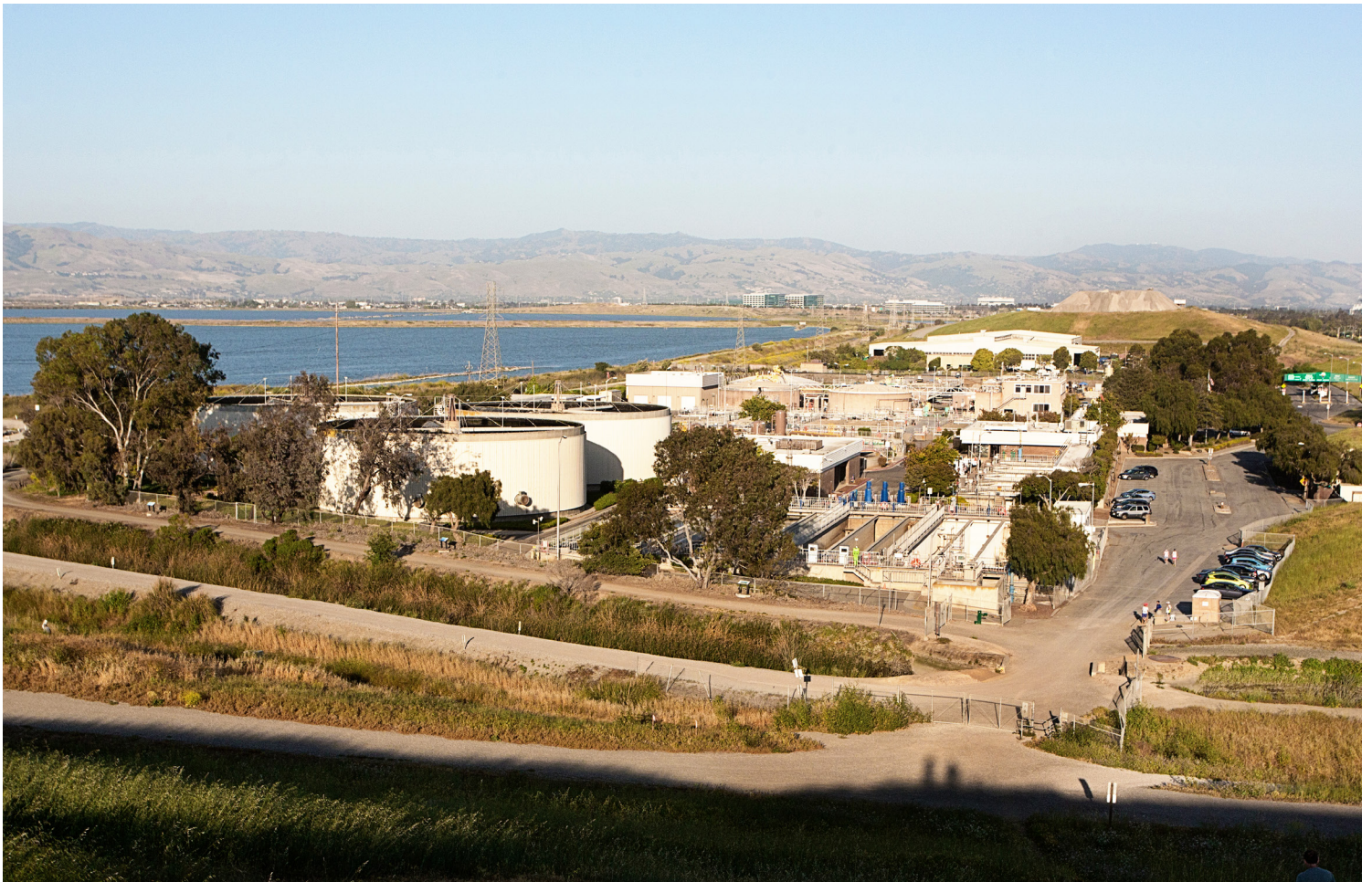
Sunnyvale's Water Pollution Control Plant located next to the San Francisco Bay
