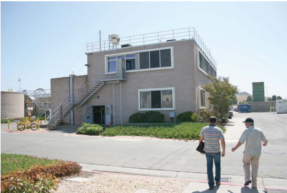
Large Meeting Room - Undersized for occupant load and inaccessible
