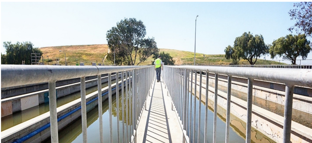
Figure 8: Chlorine Contact Tanks disinfection process
