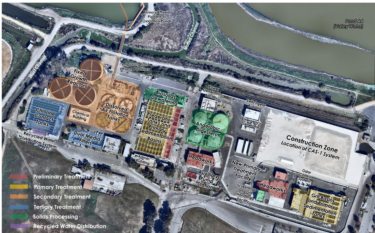
Figure 3: Aerial photo of WPCP and its various treatment processes
