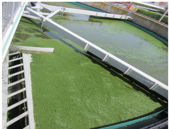
Figure 8: Algae being skimmed off the surface of wastewater in a Dissolved Air Flotation Tank
