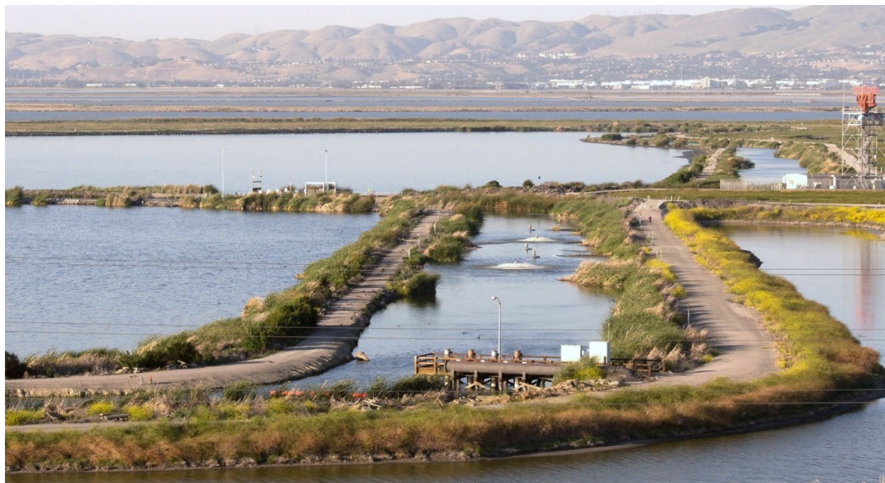
Figure 6: Oxidation Ponds, including the return/distribution channel, Pond Effluent Pump Station, and surface aerators
