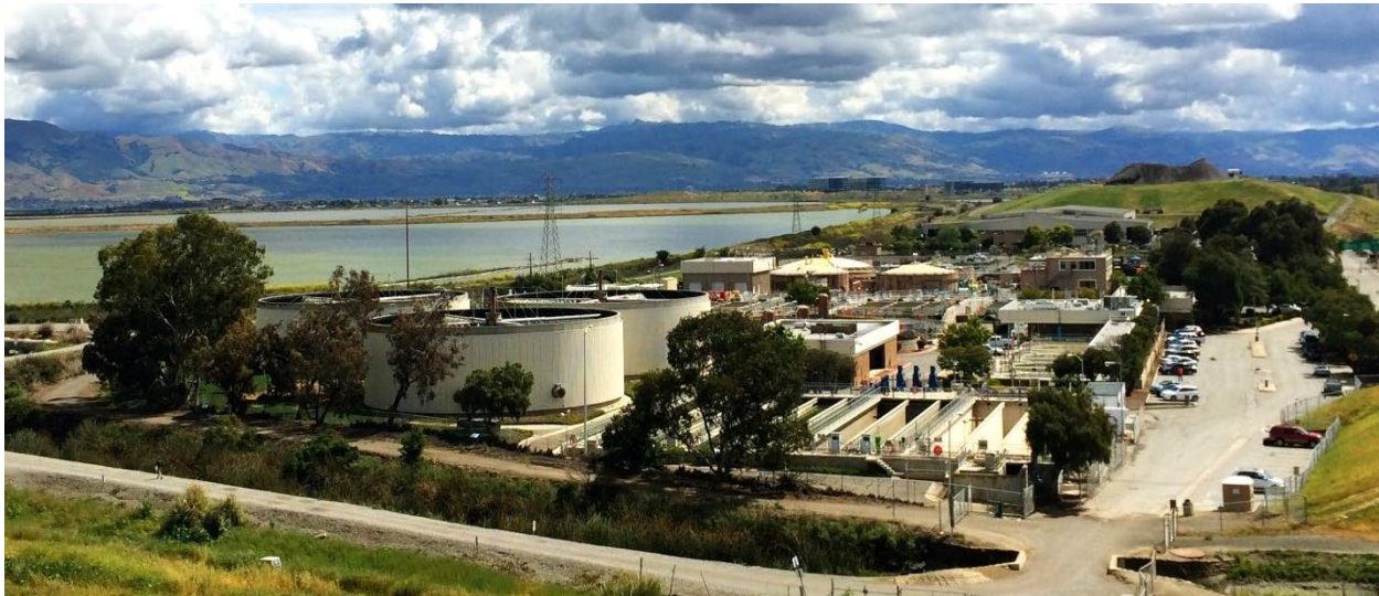
Figure 30: View of the WPCP Looking East
