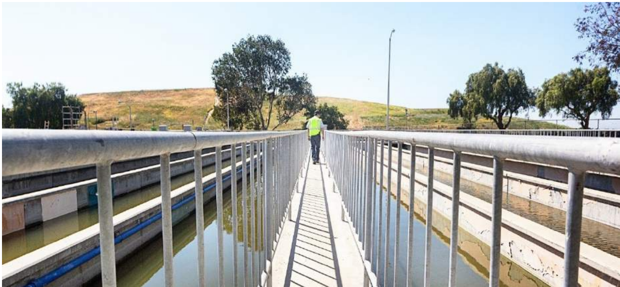
Figure 10: Wastewater being disinfected in the Chlorine Contact Tanks prior to discharge into Moffett Channel
