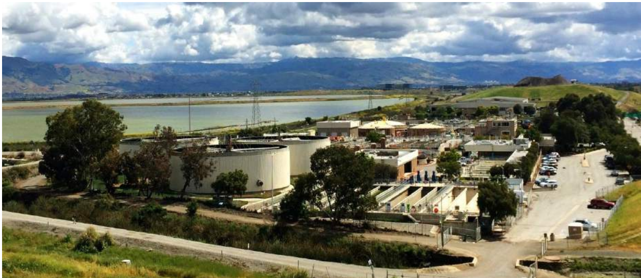
Figure 32: View of WPCP looking east
