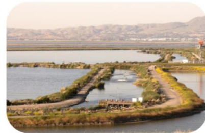
Oxidation Pond Levees
