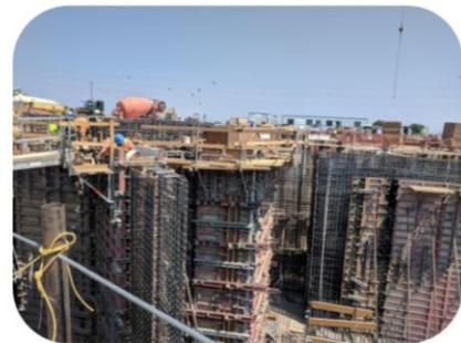
Construction of new Primary Facilities
