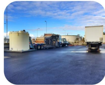
New Synagro Dewatering Area
