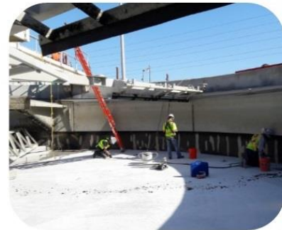
Contractor assessing an Air Floatation Tank
