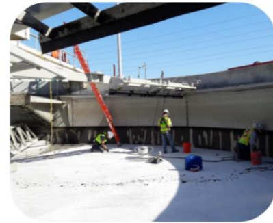
Contractor assessing an Air Flotation Tank
