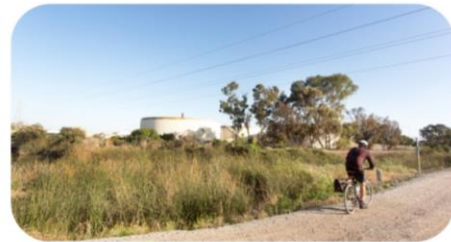
Partial Area of Bay Trail Levee Enhancements
