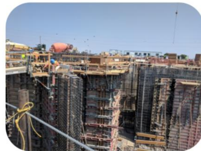
Construction of new Primary Facilities
