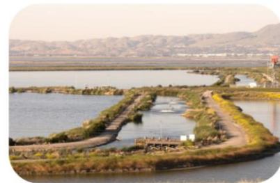
Oxidation Pond Levees
