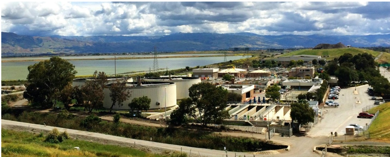
Figure 32: View of WPCP looking east
