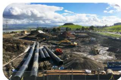
Construction of new Primary Facilities
