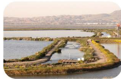
Oxidation Pond Levees
