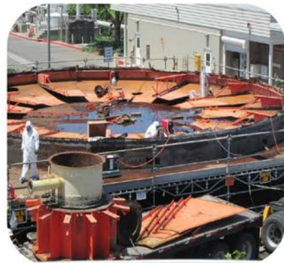
Contractors working on a digester lid
