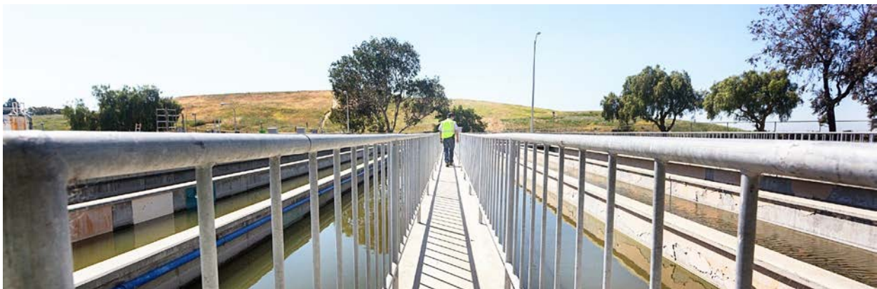
Figure 10: Wastewater being disinfected in the Chlorine Contact Tanks prior to discharge into Moffett Channel
