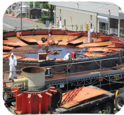
Contractors working on a digester lid
