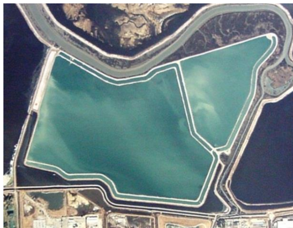
Figure 6: Aerial photo of the Oxidation Ponds
