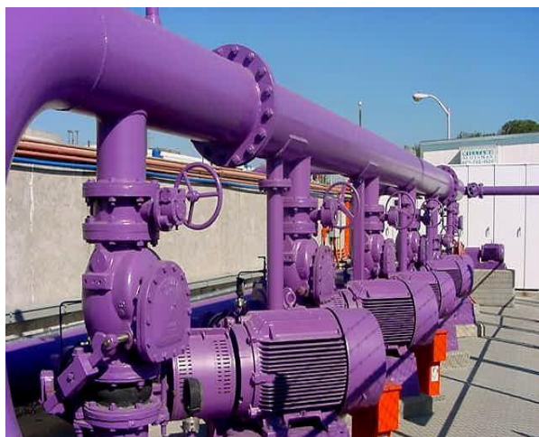
Figure 12: WPCP Recycled Water distribution piping
