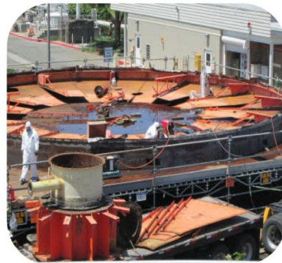
Contractors working on a digester lid in May 2014
