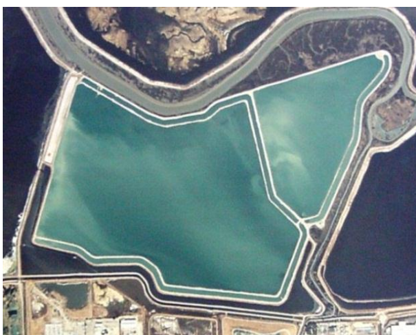
Figure 6: Aerial photo of the Oxidation Ponds
