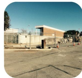
Construction area for new Recycled Water pumping station.
