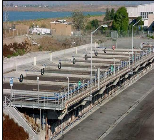
Figure 12: Dewatering Beds Treating Biosolids Prior to being hauled Off-Site for Beneficial Use
