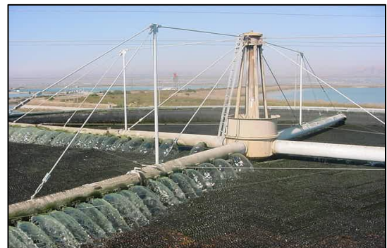
Figure 6: Rotating Arm of FGR Distributing Pond Effluent over Plastic Growth Media
