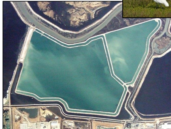
Figure 5: Bottom: Aerial Photo of 440 Acres of Facultative Oxidation Ponds. Top: Snowy Egret Commonly Found in and around the Oxidation Ponds
