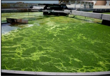
Figure 7: Algae being skimmed off the Surface of FGR Effluent Wastewater in a DAFT
