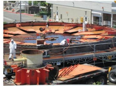
Contractors working on a digester lid in May 2014
